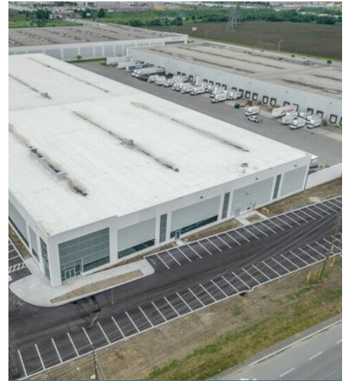
GOREWAY PHASE III, BRAMPTON, ON
