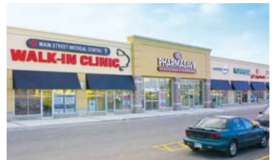
Wanless Centre, Brampton, Ontario
