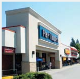
Poco Place, Port Coquitlam (C.-B.)
