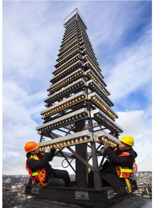
The beacon being retrofitted with LEDs
