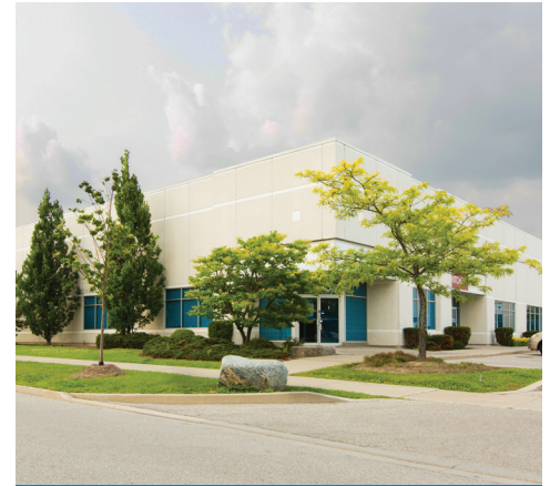
LAIRD BUSINESS PARK, MISSISSAUGA (ONTARIO)
