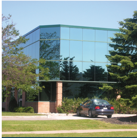
Superior Business Park, Mississauga, ON
