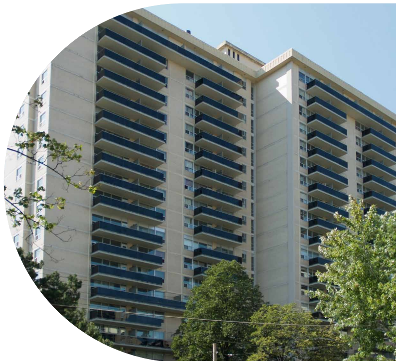
↑ Grenadier Square (40 High Park Ave & 77 Quebec Ave) (Toronto, ON)
